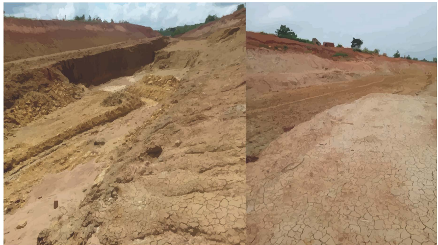
Figure 4. Slope instabilities in the study area.
