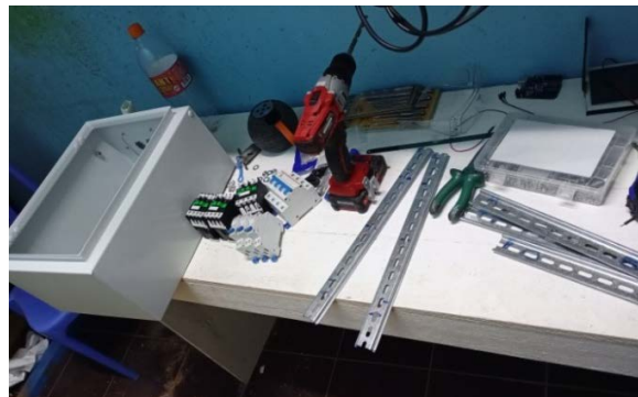
Figure 12. Drilling and cutting.
