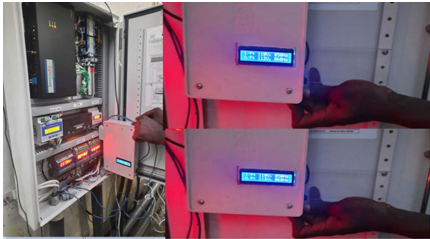
Figure 15. The setup for the implementation of 110 V/60 Hz test.
