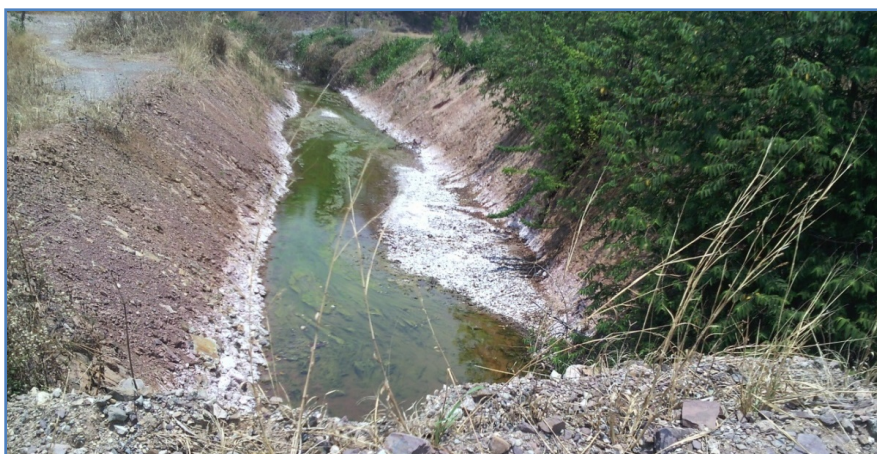
Figure 2. View of a liquid effluent drain from the Luita plant.
