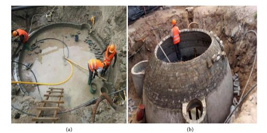
Figure 2. The design of biodigester.
