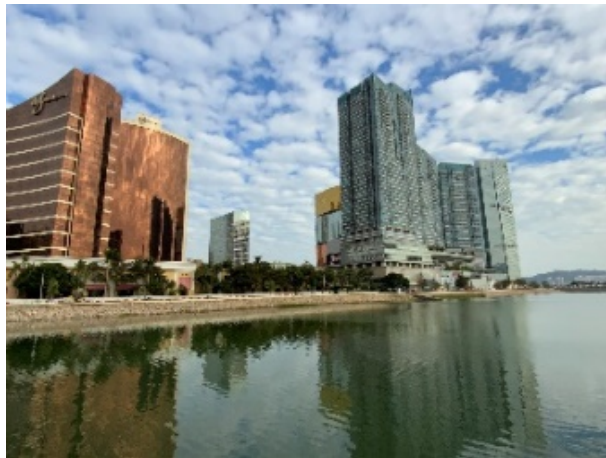
Figure 9. East bank of Nanwan Lake Area (2021) (The picture was taken by the author).
