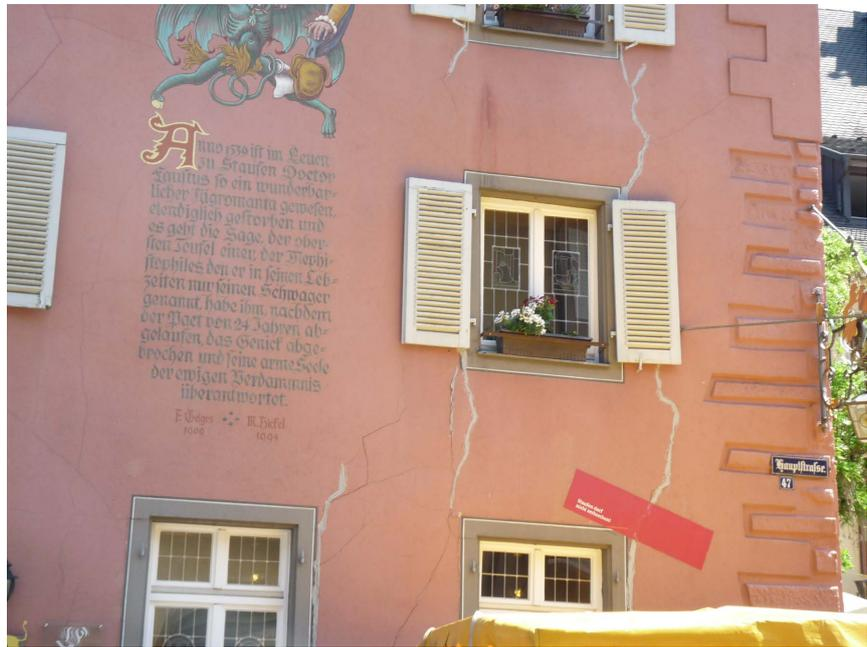
**Figure 1.** Cracks at a building in Staufen im Breisgau (Upper Rhine Graben, Germany, 2013).
