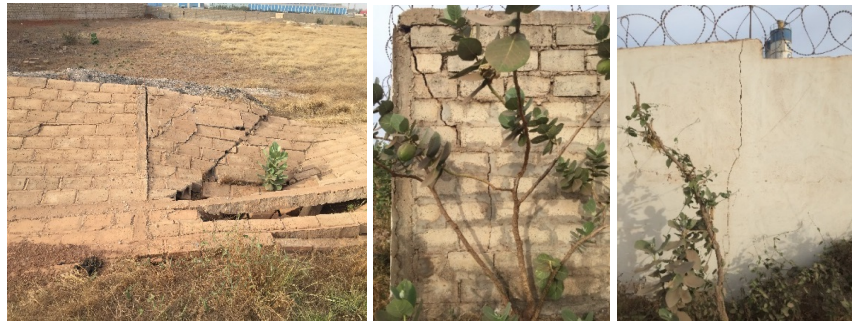
Figure 3. Disorders attributed to the shrinkage-swelling of clays near the study site.
