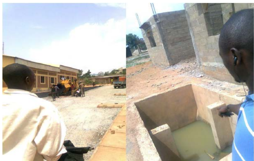
Figure 23. Construction site images in Ibadan showing their states.
