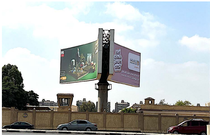
Figure 14. A street billboard constructed in a military site, 2021; the author.
