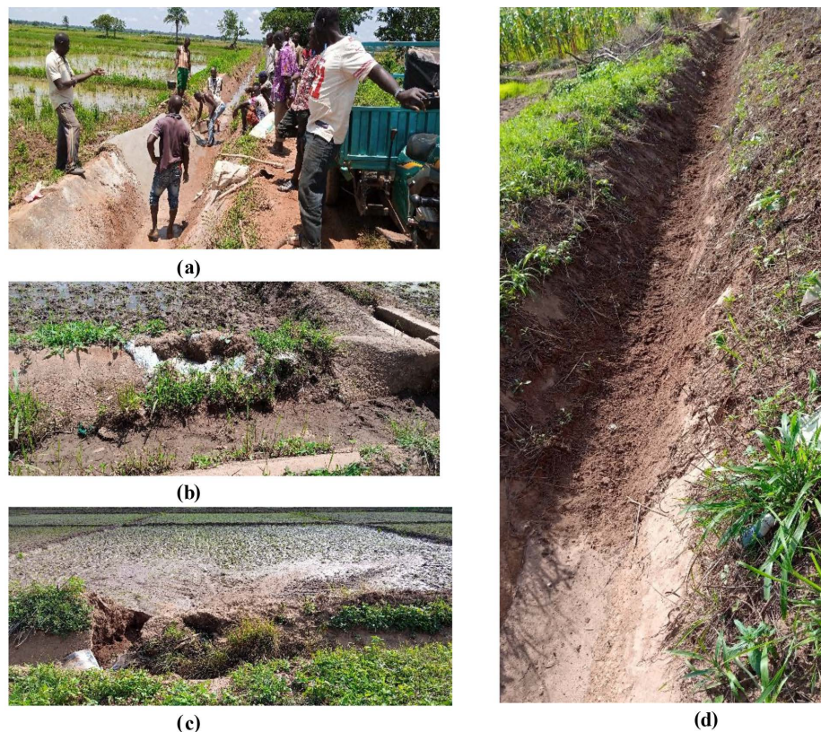
Figure 10. upkeep and maintenance operations of the canals: (a) rehabilitation of S3 by cooperative III; (b) rehabilitation of a tertiary canal by an operator; (c) rehabilitated tertiary channel which has failed; (d) tertiary canal weeded and cured.
