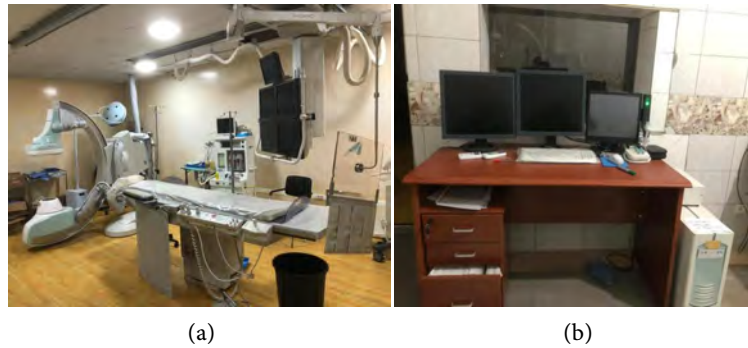
Figure 1. (a) & (b) CATH LAB 2 interventional radiology device, control room.
