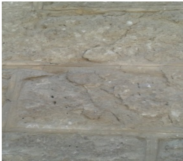
Figure 8. Effect of borrowing on limestone.
