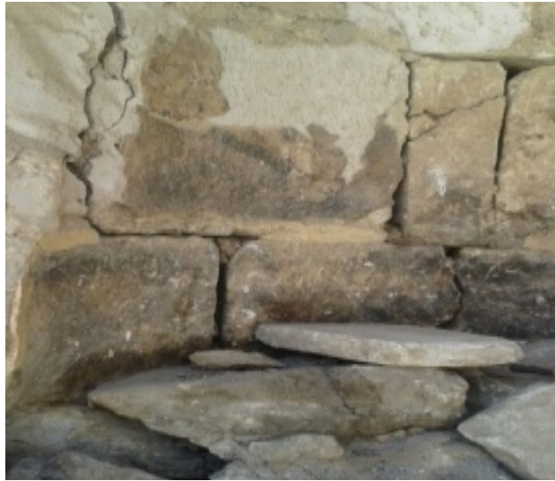
Figure 7. Loosening of stone crust.
