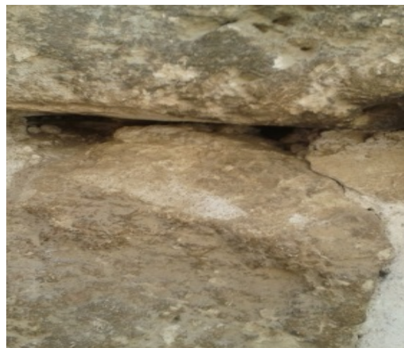
Figure 6. Detachment and salt crust on limestone surface.
