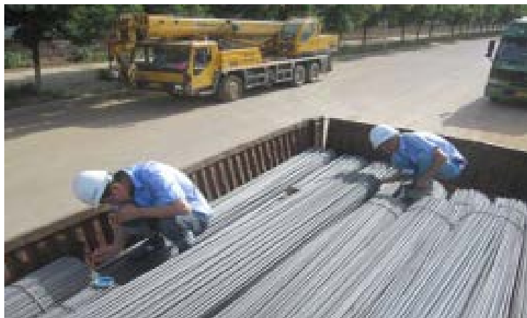
Figure 1. Manual counting of steel bars.
