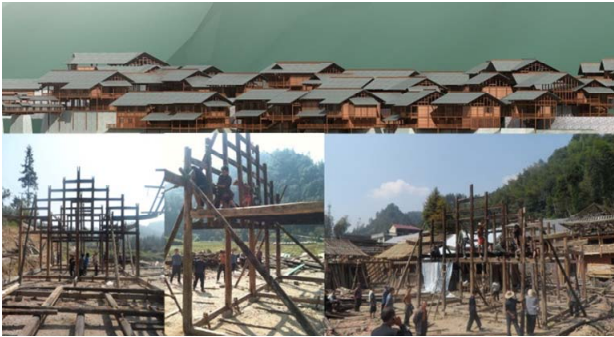
Figure 15. Directing Tujia people to build new stilted buildings using authentic traditional techniques picture by Kui Zhao, 2010.
