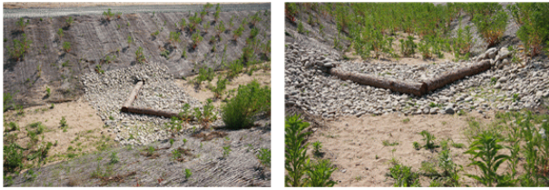
Figure 2. V-type drop structure for the verification test.
