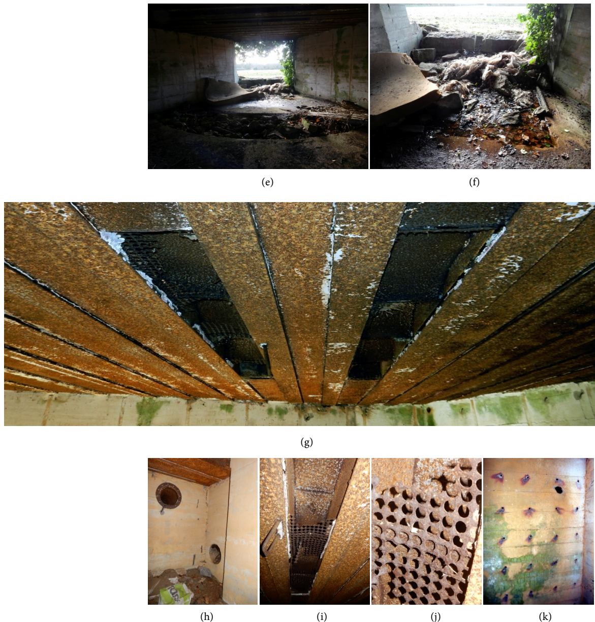
Figure 19. R 669 (3): (a) Fire room rear side aperture covered by vegetation; (b) Fire room seen from the rear side aperture; (c) Fire room front side aperture with splinter guards covered by vegetation; (d) Fire room, rear side aperture, square carriage wheel gun emplacement and arcuate gun carrier legs emplacement; (e) Square carriage wheel gun emplacement; (f) Square carriage wheel gun emplacement; (g) Fire room, metallic ceiling with gates of the combat gas extraction system; (h) Combat gas extraction system room; (i) Fire room, metallic ceiling with gun lifting joint and gates of the combat gas extraction system; (j) Grid of a gate of the combat gas extraction system; (k) Fire room rear side aperture, holes in the concrete wall.
