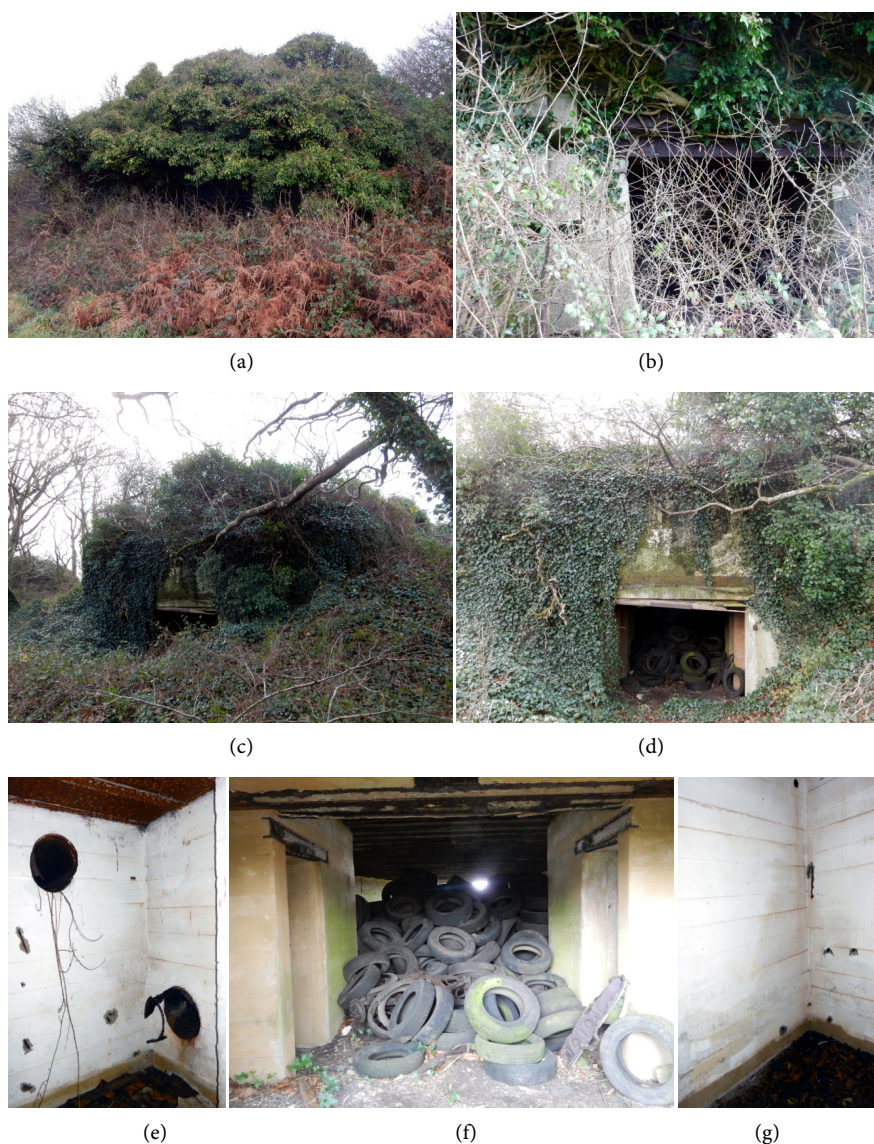
Figure 5. Stp Re 80-R 669 (2) : (a) Front side covered by vegetation; (b) Fire room front aperture; (c) Rear side covered by vegetation; (d) Fire room rear side aperture; (e) Combat gas extraction system room; (f) Fire room, on the left side entrance of the combat gas extraction system room, on the right entrance of the ammunition room; (g) Ammunition room.
