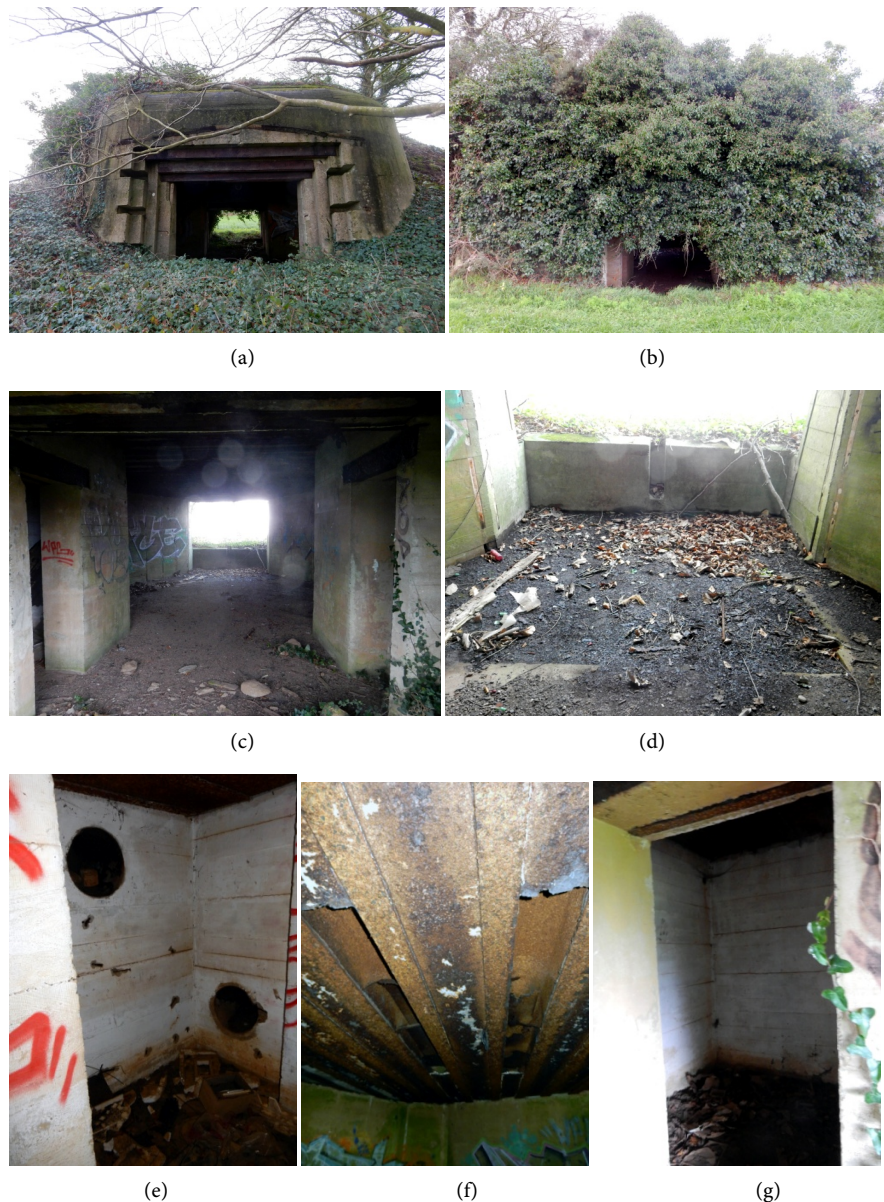
Figure 4. Stp Re 80-R 669 (1) : (a) Fire room front side aperture with splinter guards; (b) Fire room rear side aperture partially covered by vegetation; (c) Fire room, on the left side, entrance of the combat gas extraction system room, on the right side entrance of the ammunition room; (d) Fire room front side aperture and square carriage wheel gun emplacement; (e) Combat gas extraction system room; (f) Fire room, metal ceiling with gates of the combat gas extraction system; (g) Ammunition room.
