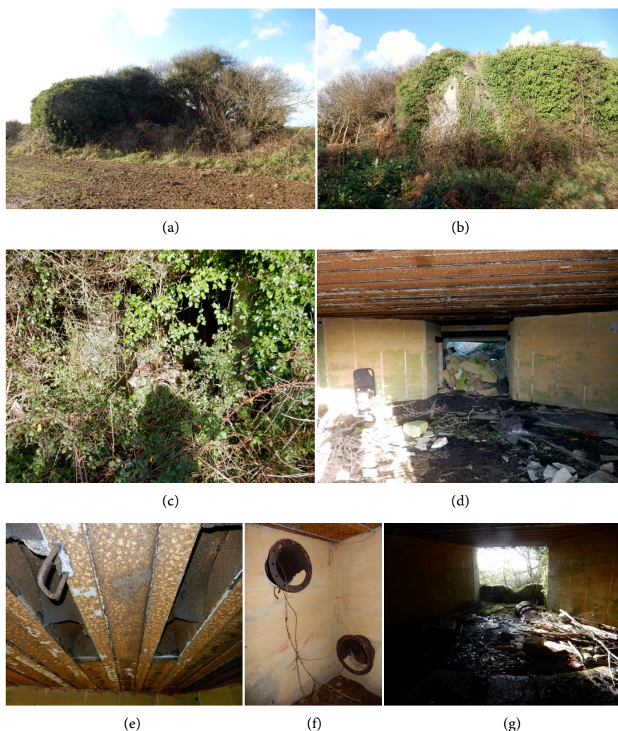
Figure 20. Stp Re 77-R 669 (4) : (a)-(b) External structure covered by vegetation; (c) Fire room front side aperture covered by vegetation; (d) Fire room, rear side aperture and arcuate gun carrier legs emplacement; (e) Fire room, metallic ceiling with gates of the combat gas extraction system and gun lifting joint; (f) Combat gas extraction system room; (g) Fire room, front side aperture and arcuate gun carrier legs emplacement.
