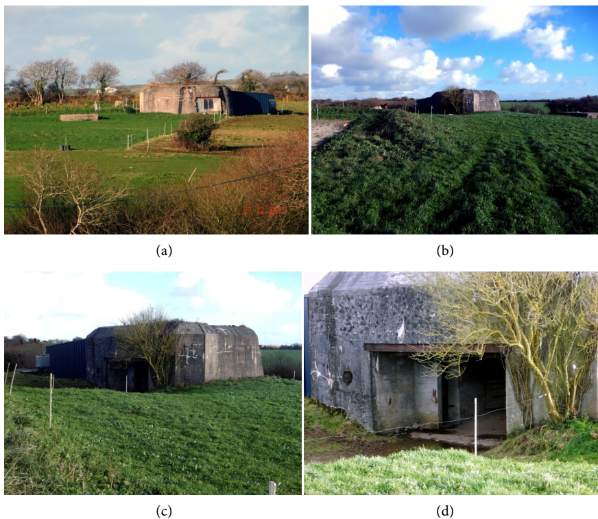
Figure 23. Stp Re 79 : (a) R 669 (3) front side, on the left Vf (1); (b) R 669 (3) rear side; (c) R 669 (3) rear side, on the left modern agricultural shed; (d) R 669 (3), fire room rear aperture with entrance of the combat gas extraction system room, on the left exhausted combat gas pipe.
