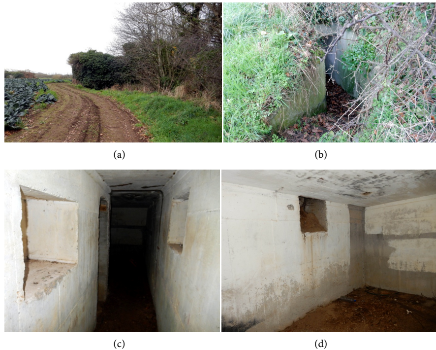
Figure 14. Stp Re 77-Vf(6) : (a) Access road; (b) Labyrinth entrance, (c) Internal corridor with niches, (d) Internal room with emergency exit.
