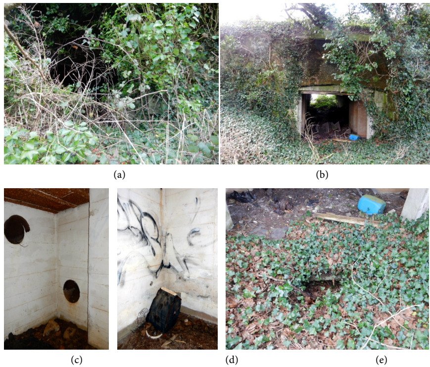
Figure 6. Stp Re 80-Re 669 (3): (a) Fire room front side aperture covered by vegetation; (b) Fire room rear side aperture; (c) Combat gas extraction system room; (d) Ammunition room, on the floor, abandoned, a washing machine drum; (e) Trench floor, bore of the drainage system.
