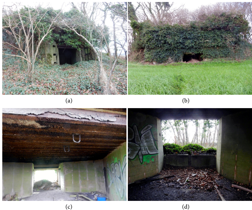
Figure 6. Stp Re 80-Re 669 (3): (a) Fire room front side aperture covered by vegetation; (b) Fire room rear side aperture; (c) Combat gas extraction system room; (d) Ammunition room, on the floor, abandoned, a washing machine drum; (e) Trench floor, bore of the drainage system.
