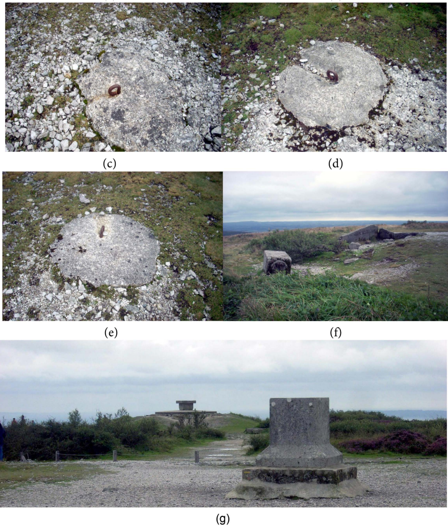
Figure 5. Menez-Hom, hill top—(a) concrete block covered by the vegetation; (b) concrete blocks of a rectangular support; (c)–(e) antenna anchoring bases; (f) damaged concrete wall and reversed concrete block; (g) geodetic stone, in the foreground the orientation table.
