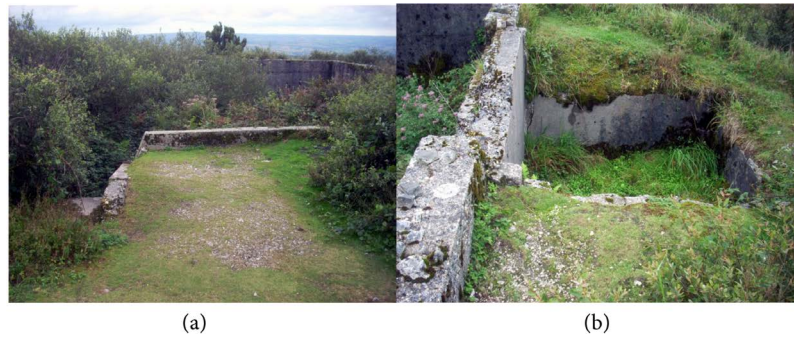
Figure 8. Menez-Hom hill, barrack emplacement 8—(a) descending stair and cavity invaded by the vegetation; (b) displaced side portion and pit at the exterior of the west side.
