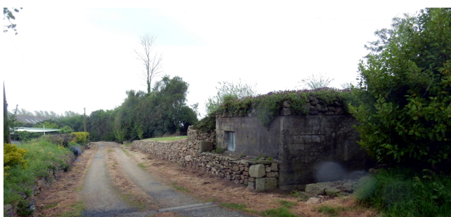
Figure 15. Le Veleury—La Metairie St.P. Av 55—one room bunker 2. partially buried in the terrain.
