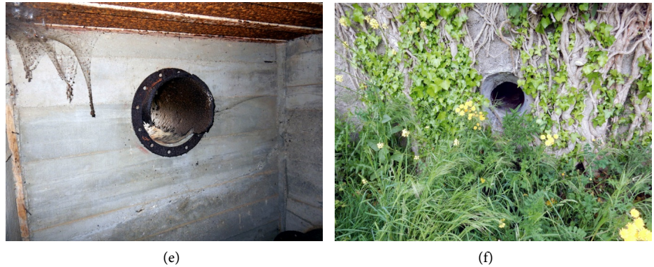
Figure 30. Le Veleury—La Metairie St.P. Av 55—H671 7.—(a) rear side aperture, niche and frame of the armoured door; (b) ammunition room; (c) fire room, floor covered with terrain, metallic ceiling with joint for gun lifting; (d) fire room, combat gas extraction conduit; (e) combat gas extraction system room, conduit; (f) niche of the exhausted combat gas conduit.
