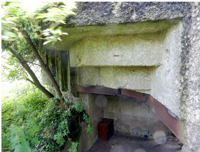
Figure 20. Le Veleury—La Metairie St.P. Av 55—H671 bunker 3.—fire room front side aperture with splinter guards.
