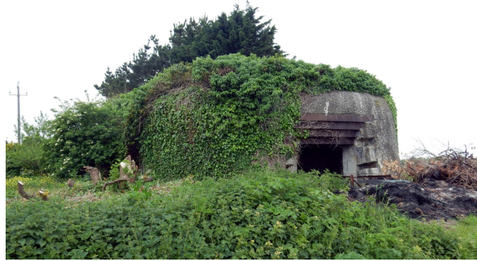
Figure 38. Kerbreslauen St.P. Av 82 “Unstrut”—H669 3. fire room front side aperture with splinter guards.
