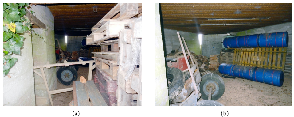
Figure 11. Rumadiou St.P. Av 59—R6693.—(a) fire room, on the left entrance of the combat gas extraction system room; (b) fire room, walled front side aperture, metallic ceiling with gates of the combat gas extraction system and joints for the gun lifting.
