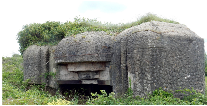
Figure 27. Le Veleury—La Metairie St.P. Av 55—H671 6.—fire room front side aperture with splinter guards and ashlar camouflage.
