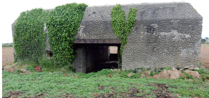
Figure 42. Kerbreslauen St.P. Av 82 “Unstrut”—H669 4.—rear side with aperture of the fire room, niche of the exhausted combat gas conduit and ashlar camouflage.
