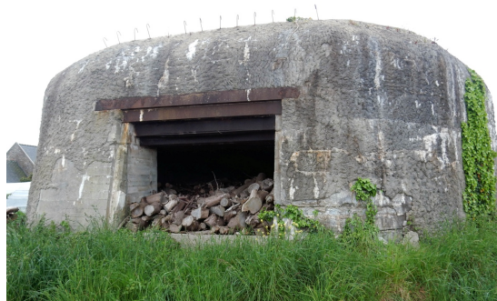
Figure 35. Kerbreslauen St.P. Av 82 “Unstrut”—H669 1., fire room front side aperture with splinter guards, ashlar camouflage, on the coverage net camouflage supports.
