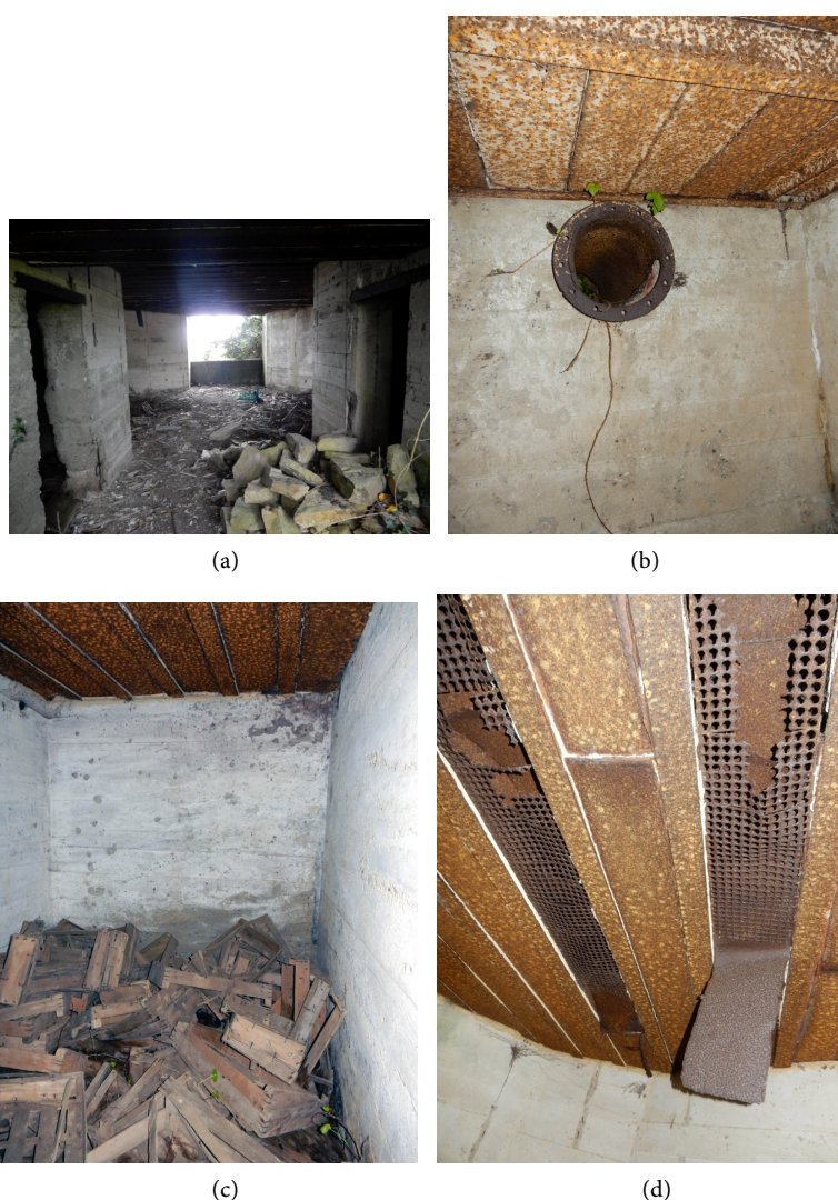
Figure 37. Kerbreslauen St.P. Av 82 "Unstrut"—H669 2.—(a) fire room, rear side aperture, on the left, combat gas extraction system room entrance, on the right, ammunition room entrance; (b) combat gas extraction system room, metallic ceiling and combat gas extraction system conduit; (c) ammunition room; (d) fire room, gates of the combat gas extraction system.
