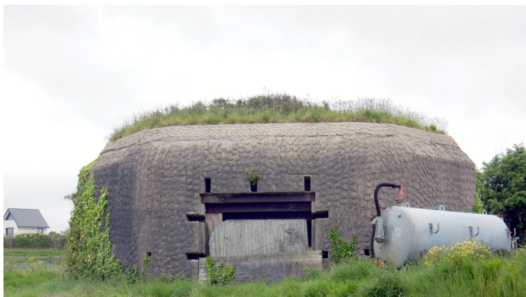
Figure 12. Rumadiou St.P. Av 59—H669 3., fire room front side aperture with splinter guards and ashlar camouflage.
