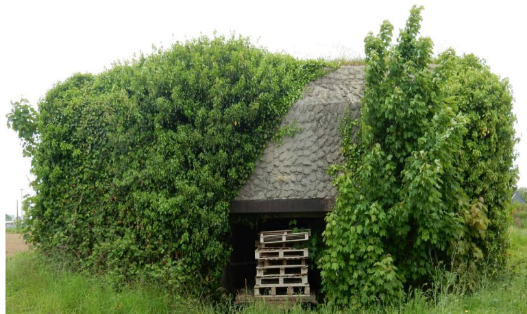
Figure 10. Rumadiou St.P. Av 59—R669 3., rear side covered by vegetation and rear side aperture of the fire room.
