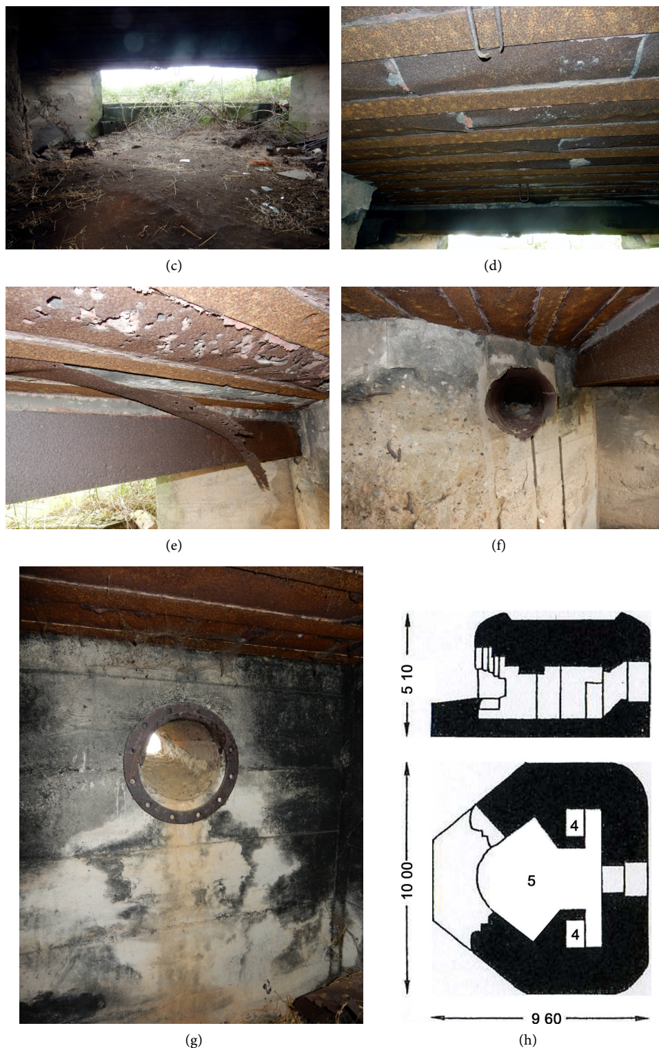
Figure 26. Le Veleury—La Metairie St.P. Av 55—H671 6.—(a) rear side aperture, niche and armored door frame of the fire room; (b) ammunition room; (c) fire room, floor covered with terrain; (d) fire room, metallic ceiling with broken joint for gun lifting; (e) fire room, metallic ceiling, details; (f) fire room, combat gas extraction conduit; (g) combat gas extraction system room, combat gas extraction system conduit; (h) H671 plan: 4. ammunition room, 5. fire room.
