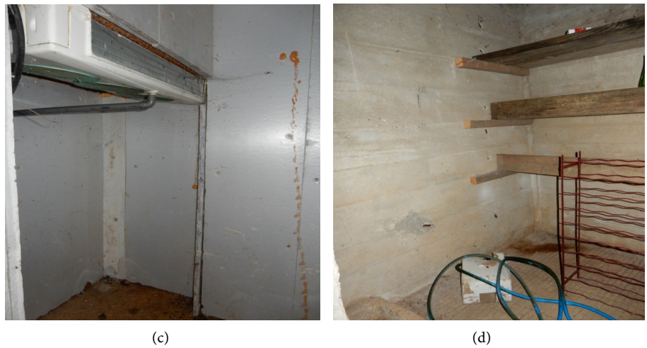
Figure 9. Rumadiou St.P. Av 59—R669 2.—(a) niche of the exhausted combat gas conduit, (b) walled front side aperture of the fire room and metallic ceiling with two joints for gun lifting, (c) combat gas extraction system room, (d) ammunition room.
