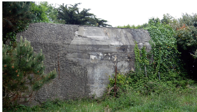
Figure 36. Kerbreslauen St.P. Av 82 “Unstrut”—H669 2., lateral side covered by the vegetation and ashlar camouflage.
