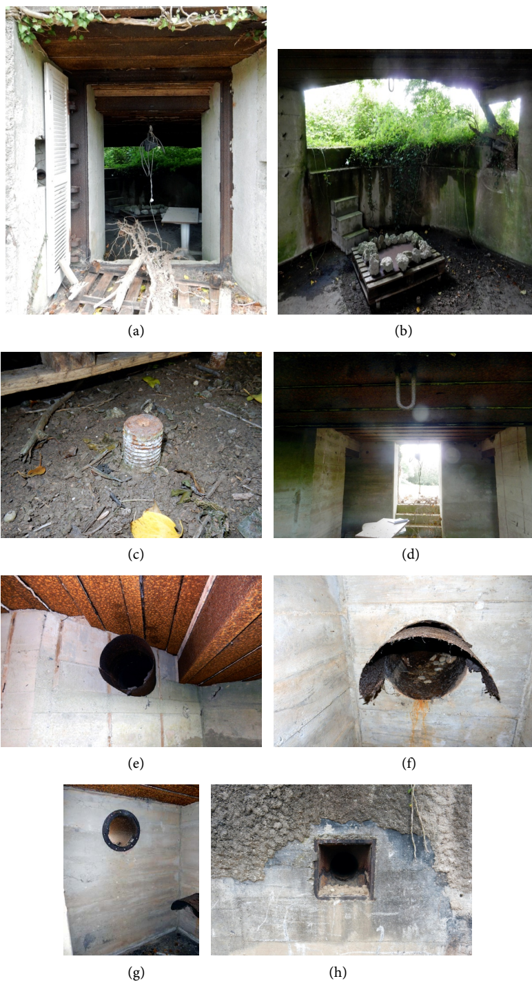
Figure 19. Le Veleury—La Metairie St.P. Av 55—H671 bunker 3.—(a) rear side aperture, niche and frame of the armored door; (b) fire room, front side aperture, pallet covering the fixation points of the gun mount; (c) fire room, fixation points of the gun mount; (d) fire room, rear side aperture, on the left, ammunition room entrance, on the right, combat gas extraction system room entrance, on the ceiling, joint for gun lifting; (e) fire room, combat gas extraction conduit; (f) combat gas extraction system room, combat gas extraction system conduit; (g) combat gas extraction system room, metallic ceiling and combat gas extraction system conduits; (h) niche of the exhausted combat gas conduit.
