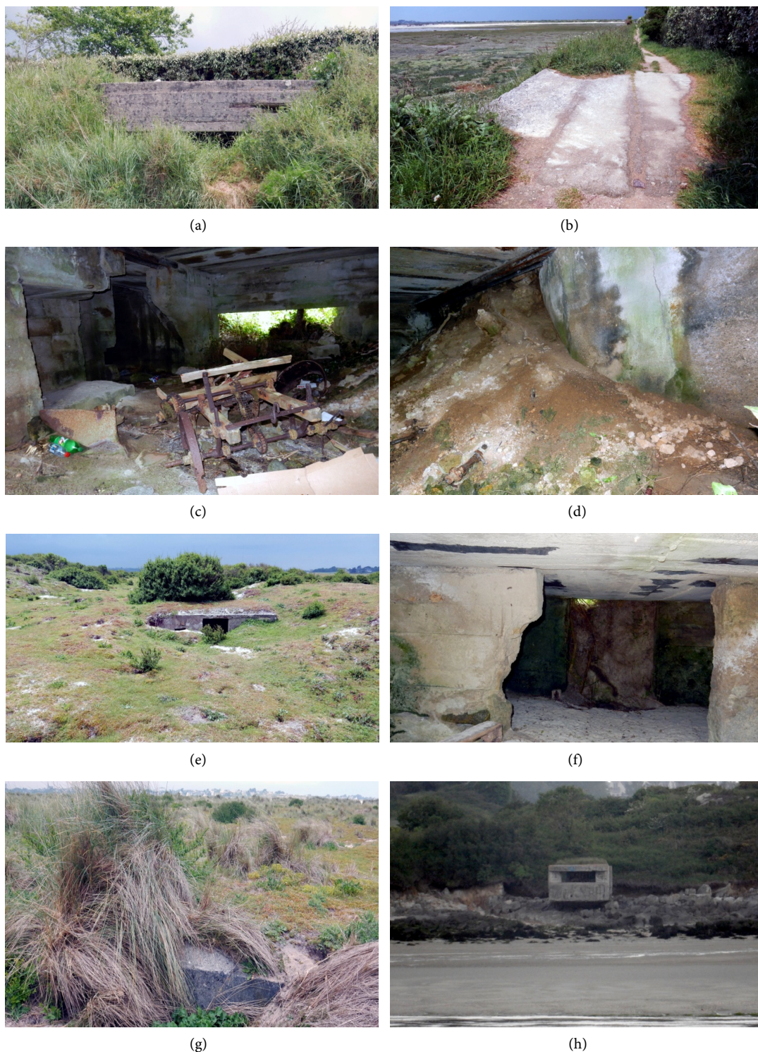
Figure 2. Close defence line—(a) bunker a., front side aperture of the fire room, (b) bunker a., concrete coverage, (c) bunker a., fire room, on the left side niche for turning the gun and possible entrance to the ammunition room, on the right side gun entrance aperture, (d) fire room filled with sand and debris, (e) bunker b., in the middle, rear side aperture of the fire room and on the left aperture for a machine gun, (f) bunker b., front aperture of the fire room filled with sand and debris, (g) bunker c., buried under sand and vegetation, (h) bunker d., front aperture of the fire room.
