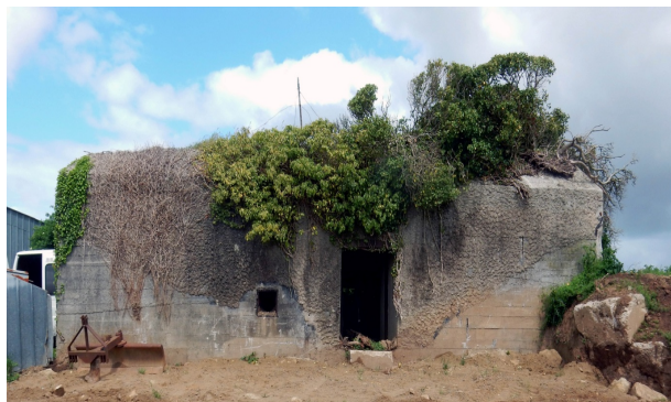
Figure 18. Le Veleury—La Metairie St.P. Av 55—H671 bunker 3.—rear side with camouflage, on the left niche of the exhausted combat gas conduit, in the middle rear side aperture of the fire room.
