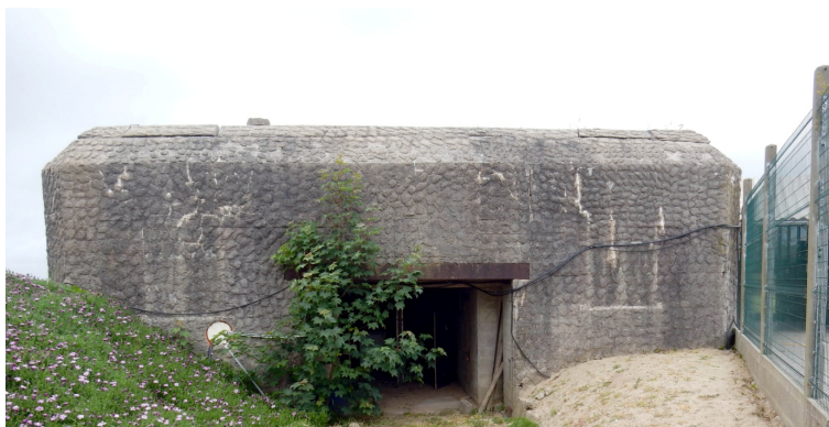
Figure 8. Rumadiou St.P. Av 59—R669 2., fire room rear side aperture and exhausted combat gas conduit niche, ashlar camouflage, on the right fence of the dog breeding.
