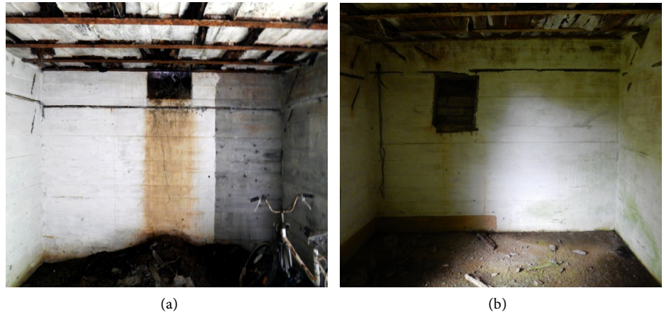
Figure 24. Le Veleury—La Metairie St.P. Av 55—one room bunker 5.—(a) wall aperture and wooden ceiling without supports of a thermal insulation system; (b) bunker interior walls, niche.
