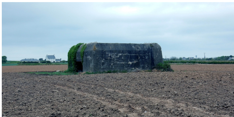
Figure 40. Kerbreslauen St.P. Av 82 “Unstrut”—H669 4.—lateral side and aperture of the fire room.
