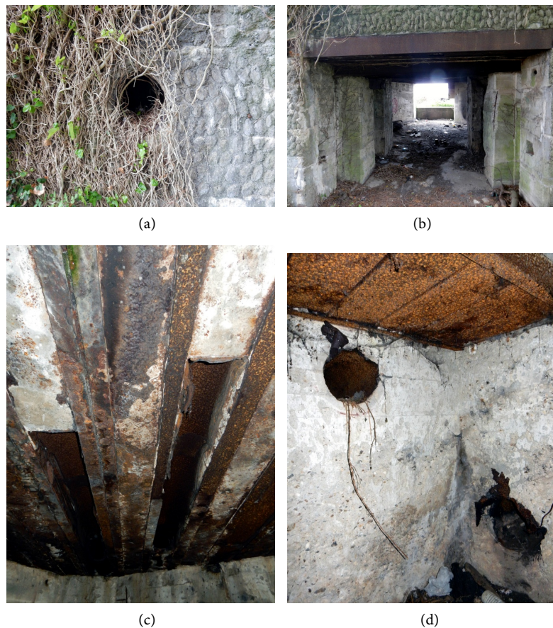
Figure 39. Kerbreslauen St.P. Av 82 “Unstrut”—H669 3.—(a) niche of the exhausted combat gas conduit fire room, rear side aperture, on the left, combat gas extraction system room entrance, on the right, ammunition room entrance; (b) combat gas extraction system room, metallic ceiling and combat gas extraction system conduits; (c) fire room, air intakes of the combat gas extraction system; (d) combat gas extraction system room, conduits.
