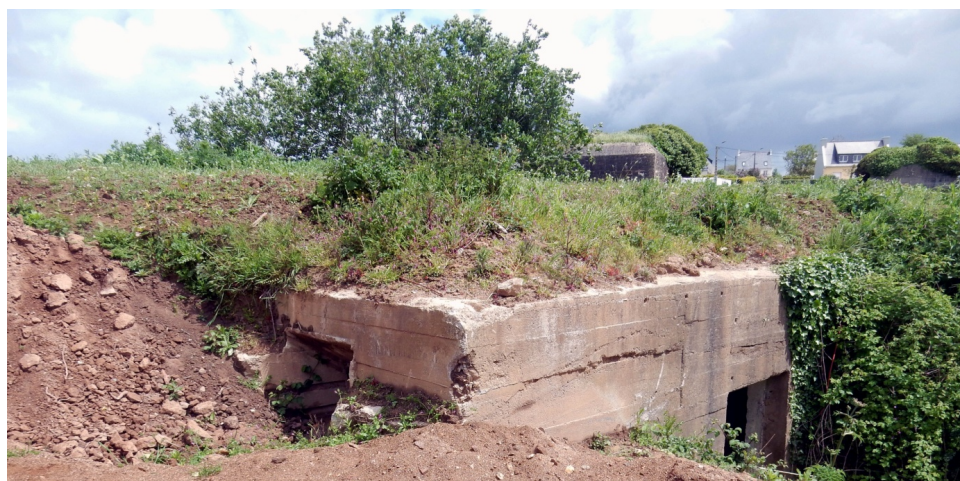
Figure 21. Le Veleury—La Metairie St.P. Av 55—one room bunker 4.—on the left wall aperture, on the right entrance.
