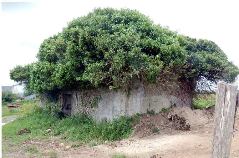
Figure 29. Le Veleury—La Metairie St.P. Av 55—H671 7.—rear side with aperture of the fire room.
