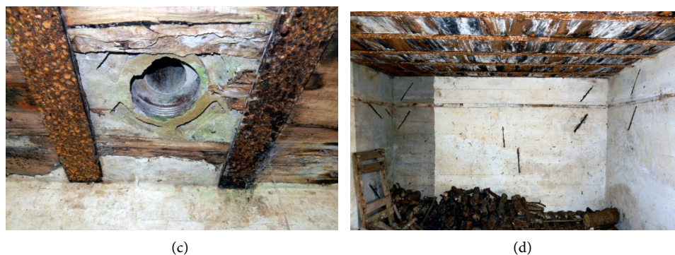
Figure 22. Le Veleury—La Metairie St.P. Av 55—one room bunker 4.—(a) wall aperture and niche, on the wall possible fixations of a thermal insulation system; (b) wooden ceiling with metallic supports; (c) chimney hole for WT80; (d) interior filled with materials.
