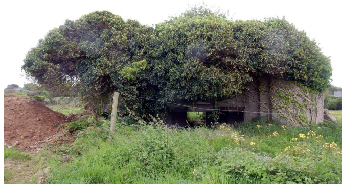
Figure 31. Le Veleury—La Metairie St.P. Av 55—H671 7.—fire room front side aperture, splinter guards covered by the vegetation, metallic ceiling with joint for gun lifting.
