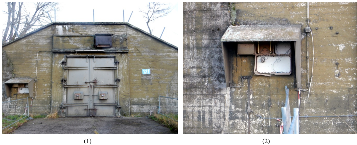
Figure 28. Airfield defense area—(1) bunker coded 121, electric control board, double door, external box of the aeration system; (2) bunker coded 121, electric control board.
