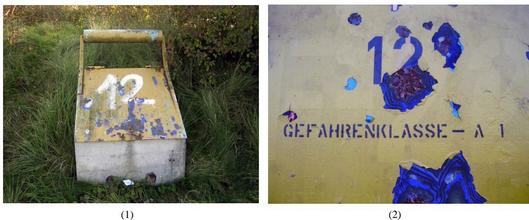
Figure 12. Airfield fuel area—(1) external, concrete control box of the underground cistern 12 (12) with closed metallic, rotatable cover and counterweight; (2) metallic, rotatable cover rear side with the indication of the hazard class A-1.
