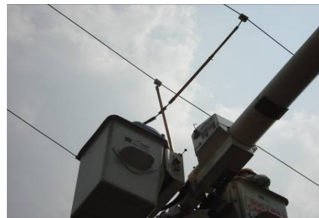
Figure 4. Insulating supporting stick in use 图 4. 支杆的现场运用
