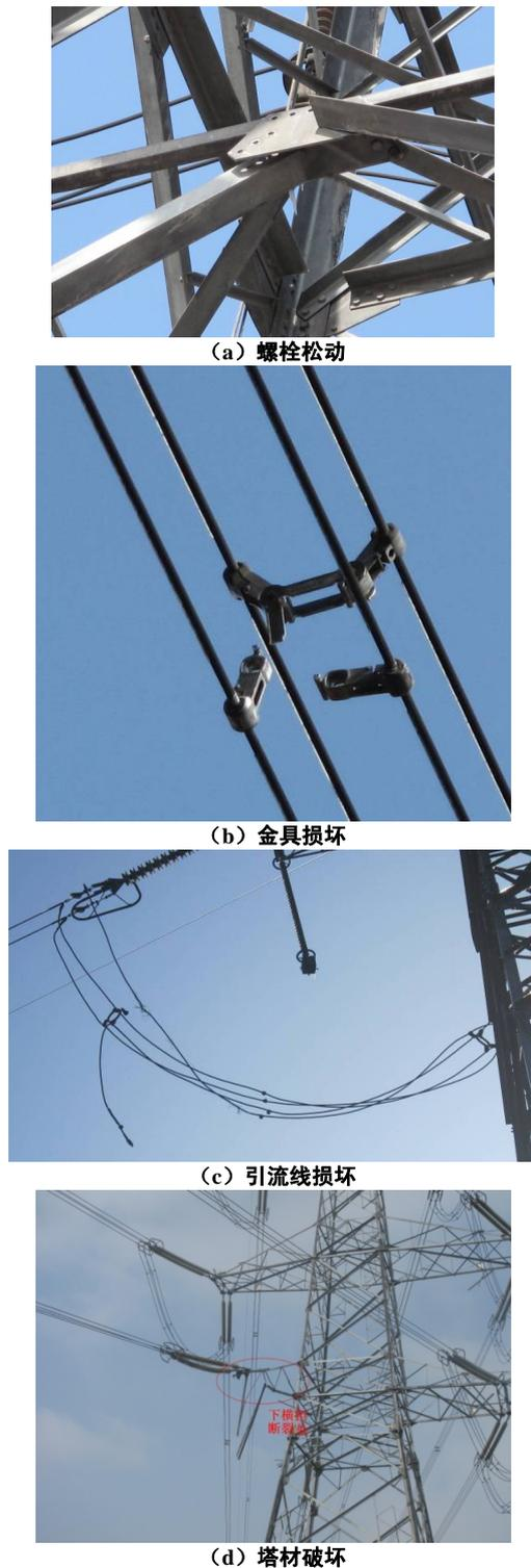
Fig 1 Damage conditions of line tower, hardware fittings and infrastructure caused by galloping
