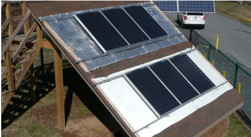
**Figure 9.** Photo of Trial 5. Upper array silver roof paint flush 3 modules, lower array white TIOCOAT™ flush 3 modules. (Refer to **Table 1** for details).
