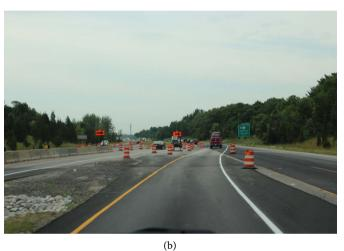
**Figure 8.** Reverse curves in the C2S work zone on I-65 (mile marker 167-176). (a) Lane divergence at mile marker 176; (b) Lane convergence at mile marker 173.
