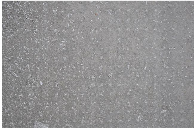
**Figure 4.** The unprotected surface of a box element in wall of the factory building (after 13 years outdoor weathering).
