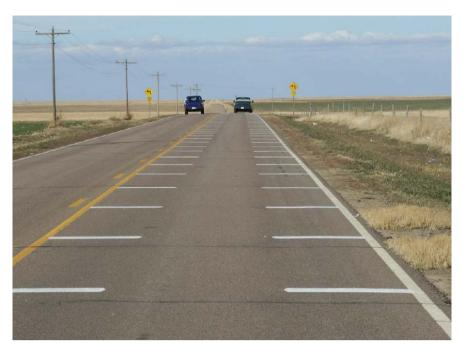
Figure 2. Picture of optical speed bars on K27 at approach to one of the curves.
