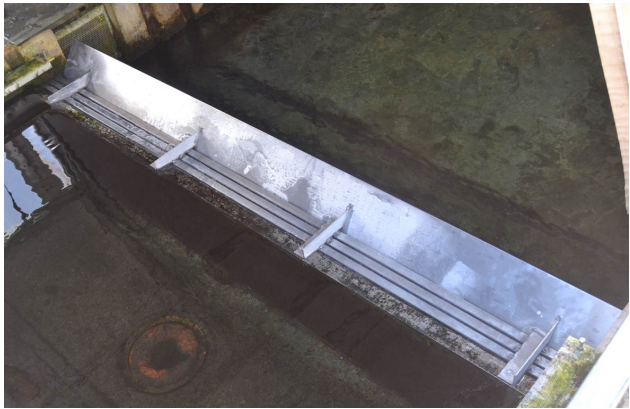
Figure 3. Image of a splash plate installed on a raceway section.
