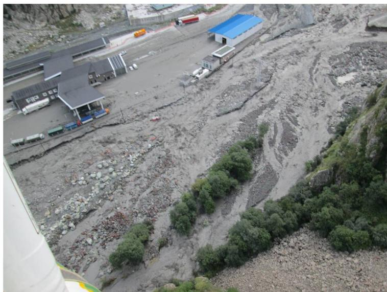
**Figure 12.** Damaged customs checkpoint building.
