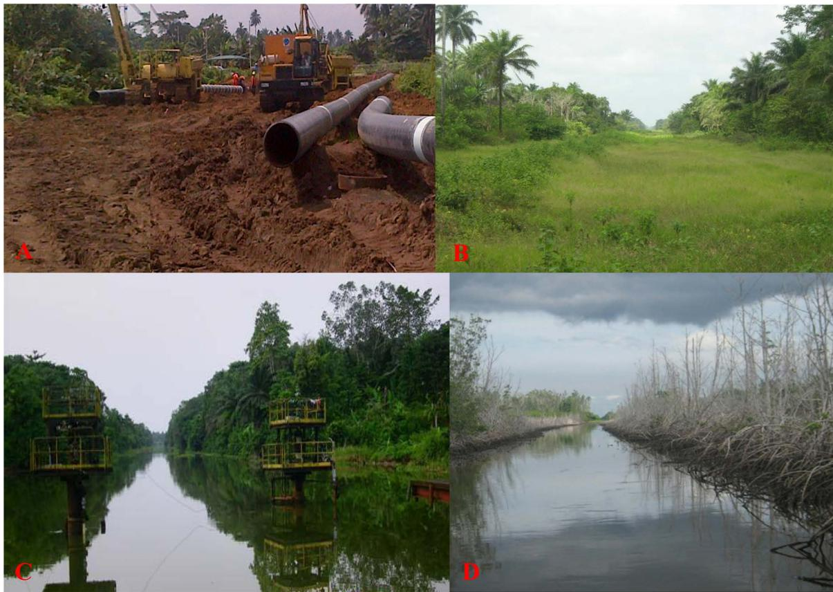
**Figure 2.** (A) Section of the 45 km pipeline under construction in moist lowland rainforest section. Notice the different earth moving equipment, excavated earth, pipes; (B)-(D) Different segments of the 120 km existing pipeline RoW ((B) is along lowland rainforest area, (C) is across freshwater swamp forest area, and (D) is through mangrove swamp forest *i.e.*, brackish water area).
