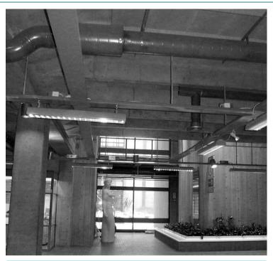
Figure 2. Example decoupling of parts and systems.
