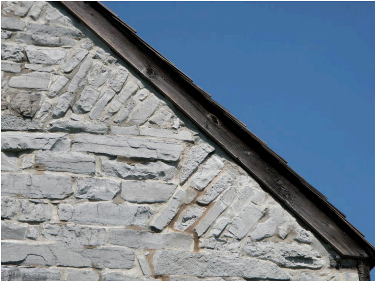
Figure 4. Dutch-influenced tumbling masonry on the south gable of Fort Klock.
