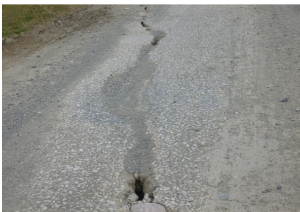
Figure 2. The effect of fault mechanism on Van-Ercis state road and its repair.
