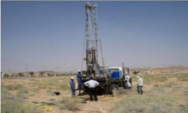
Figure 4. Acker AD II Drilling rig operating on site.
