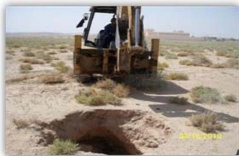
**Figure 2.** Typical sink hole close to ground surface.
