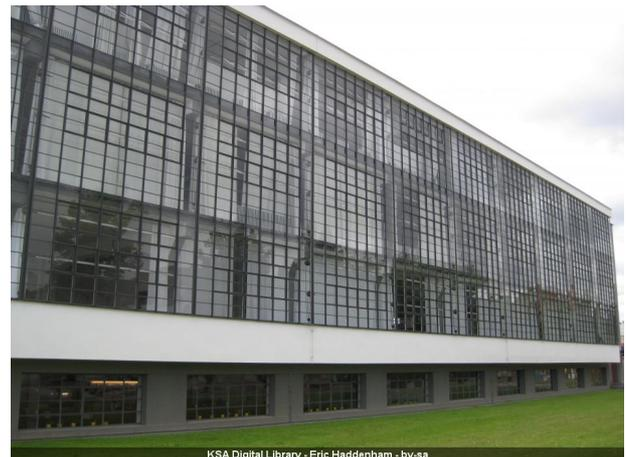
**Figure 2. Glass curtain wall of the Bauhaus Dessau, 1926 [6].**
