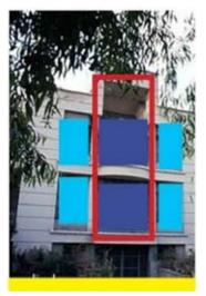
Figure 9. Façade organization with Iwan and large openings at the middle, and small openings in both sides.
