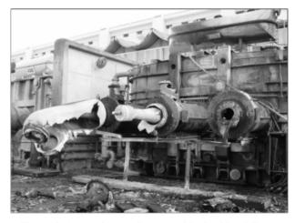
Figure 3. A transformer fire caused by bushing failure.
