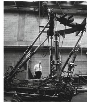
**Figure 3.** First design of an octahedral hexapod for flight simulator (courtesy of Klaus Cappel) [11].
