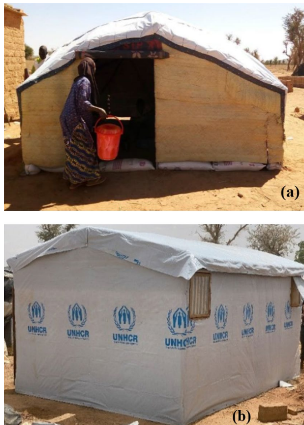
Figure 1. Standard emergency shelters: (a) Sahelian tent type [10], (b) Gabled frame type.
