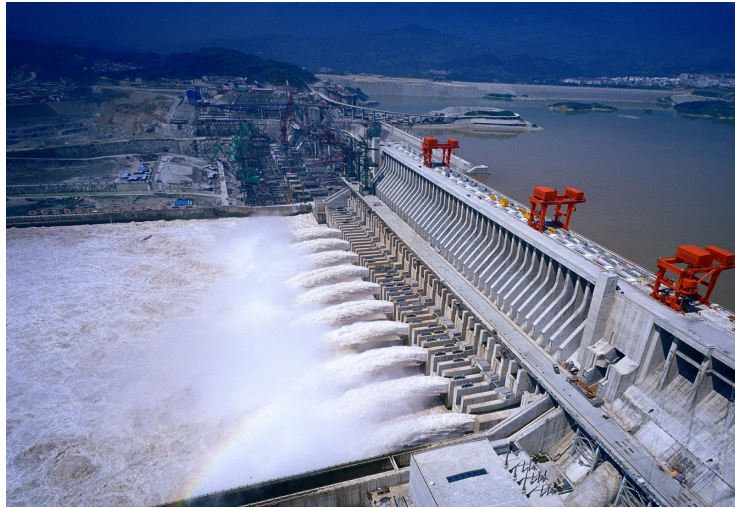
Figure 7. Electrical generation and water discharge at the Three Gorges Dam. Photo Credit: Pinterest.
