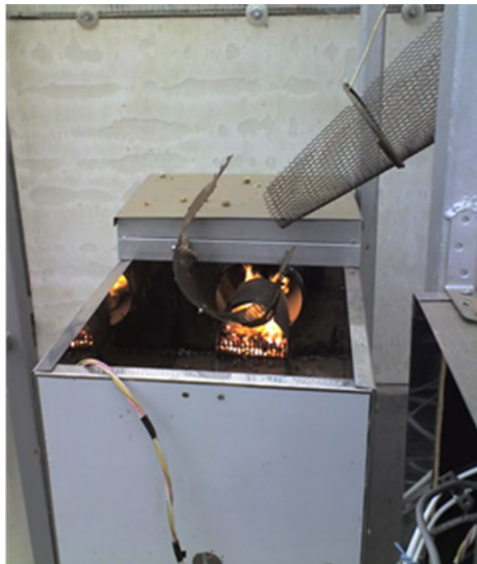
Figure 3. View of operating pellet gas burner at minimum output.
