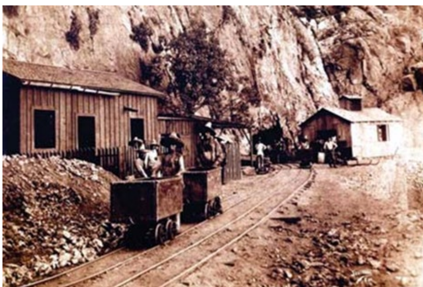
Figure 9. Steel carts and tracks for moving minerals outside the mine ( https://cienciauanl.uanl.mx/?p=4176 ).
