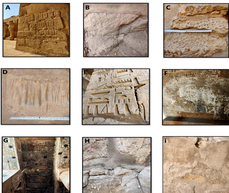
**Figure 3.** Different deterioration symptoms of Ramesses III temple (A) macro-cracks spread on the surfaces. (B) Black weathering due to Loss of scales. (C) alveolar weathering due to lose of stone material. (D) Relief. (E) Break out due to natural cause. (F) Efflorescences to light-colored crust changing the surface. (G) Microbiological colonization to dark-colored crust tracing the surface. (H) Granular disintegration into powder. (i) weathering out dependent on stone structure.
