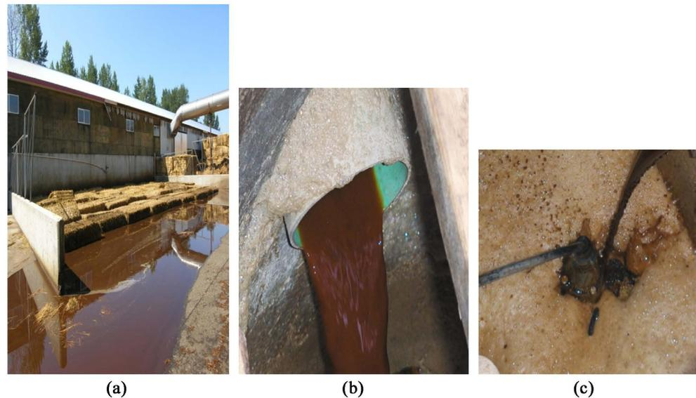
**Figure 1.** (a) It shows the soaking pit containing bales of straw and brown “goody” water. Notice the absence of bubbling on the surface of the liquid. (b) It shows entry of brown liquid from the green drain pipe into the pump chamber and the presence of beige-colored foam. (c) It highlights the role of rotation of the impeller of the pump in formation of the beige-colored foam. The beige-colored foam contains the  $H_2S$ .  $H_2S$  escapes into the chamber following breakage of the bubbles.
