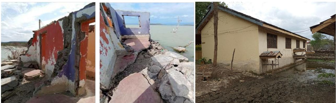
**Figure 14.** Damages on stone walled houses (Source: Author).
