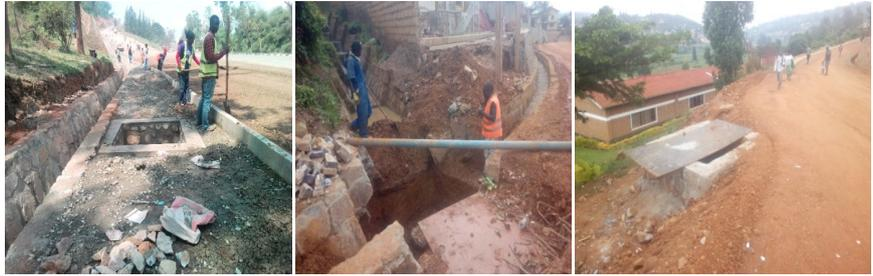
**Figure 10.** Lack of protective information for Manholes at Karama, Akagera and Agatare roads respectively.
