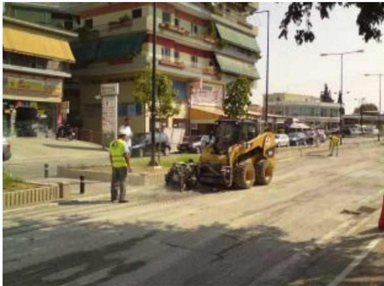
Figure 2. Removal of the old surface and cleaning at Vasilikon Street.
