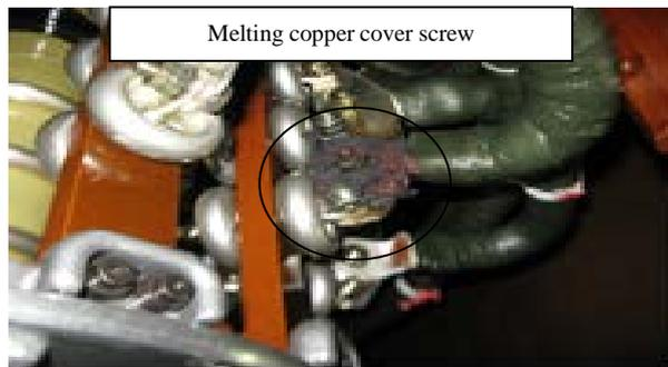
**Figure 4.** A Screw melting with copper.
