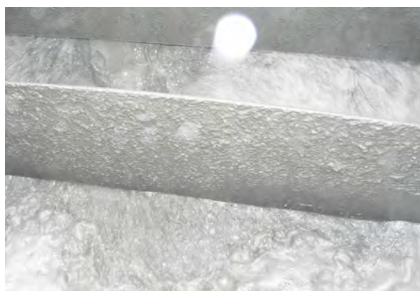
Figure 3. Placement and structure of baffles installed at top of the tailings silos to control fine size tailings overflowing
