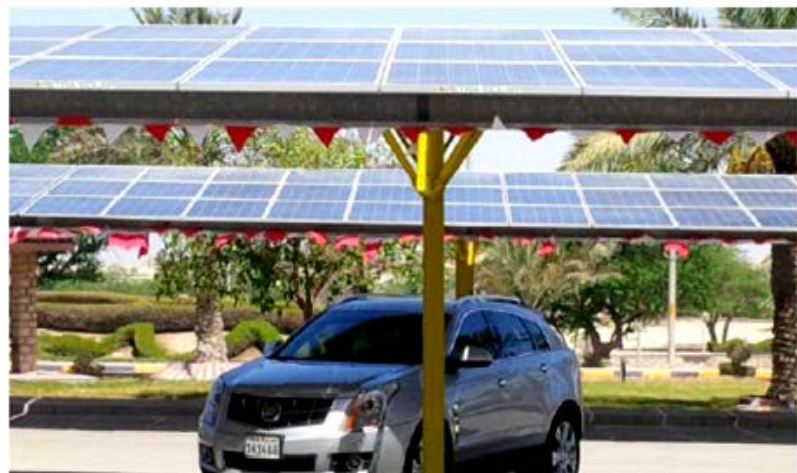
Figure 2. PV panels mounted on carports in Awali town, Kingdom of Bahrain.
