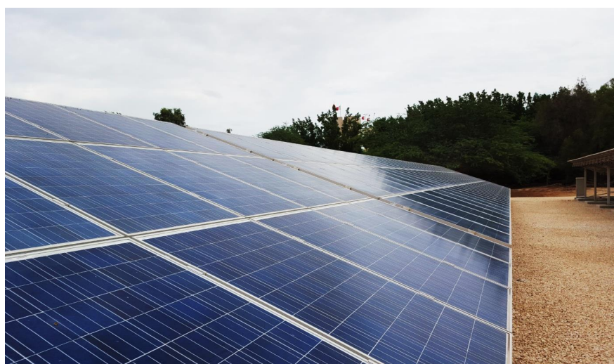
Figure 13. On the 28th of Nov. 2014 there was a heavy rain in Bahrain. The PV panels were cleaned naturally. The solar electricity from UoB panels was slightly more than the expected in this day by 10%, i.e. an extra of 233 kWh solar electricity.
