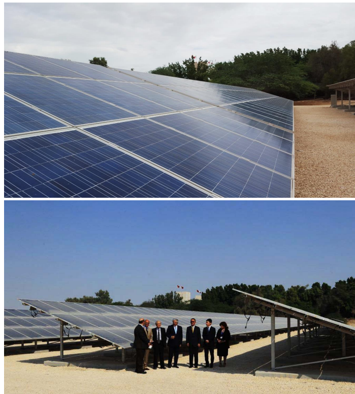
Figure 4. The 0.518 MW solar pv polycrystalline photovoltaic ground-mounted, solar-grid modules deployed at the University of Bahrain—Part of 5 MW BAPCO pilot Project in the Kingdom of Bahrain.
