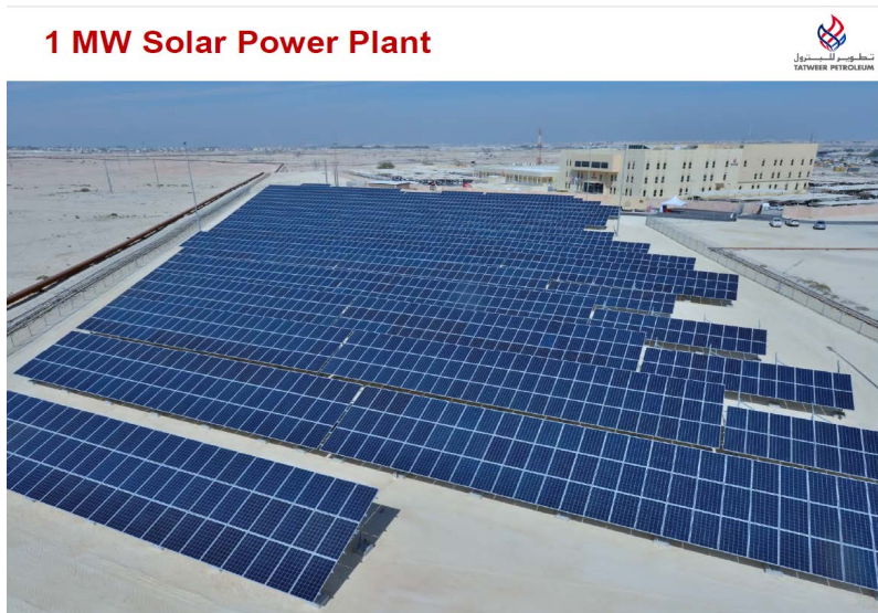
Figure 16. The 1 MW polycrystalline PV installations in Bahrain by Tatweer Petroleum. The projected started operation in Operation since 2017. The efficiency of the PV panels is 15.4% with 16 invertors @ 60 kVA. The projected was constructed in 5 months only on a land of 14,900 m 2 with PBP of 12 years.
