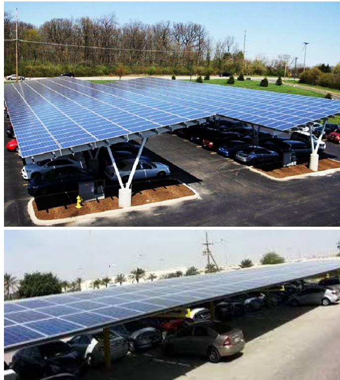
Figure 5. The refinery 2.7 MW car ports solar PV polycrystalline connected to national grid—Part of 5 MW BAPCO pilot project in the Kingdom of Bahrain.
