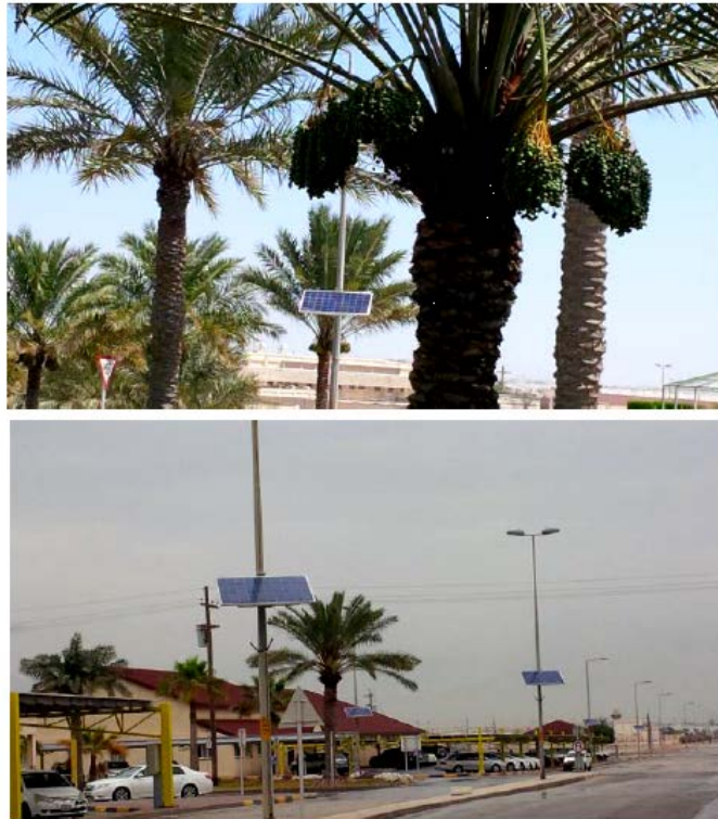
Figure 3. PV panels mounted on street light poles in Awali town, Kingdom of Bahrain.
