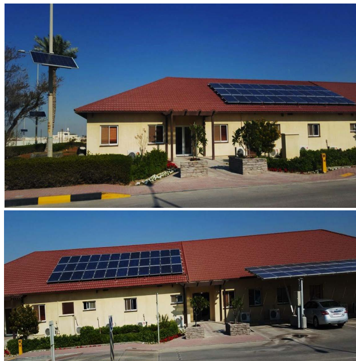
Figure 6. Sadeem Building: First BIPV in Bahrain at Bapco, Awali Town, 8.64 kW. It consists of 36 panels on the roof each has 240 Wp. The panel's orientation is 225^\circ from the North. The PV panels have tilt angle of 25^\circ . The total area of PV panels on the roof is about 60 \text{ m}^2 . Note that the latitude of Bahrain is 26.13^\circ \text{N} and the longitude is 50.8^\circ \text{E} .
