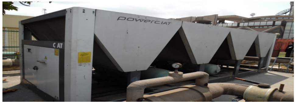
Figure 2. Cold store AQUACIATPOWER LD 1800BV standard R410A.
